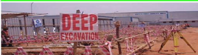
Work area Barrication
