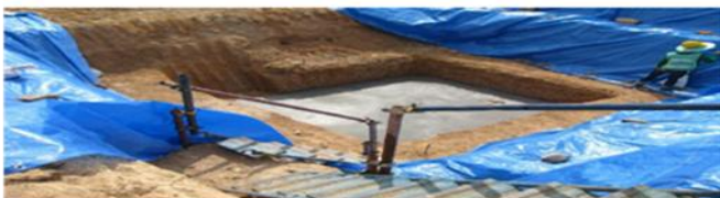
Ladder for access
