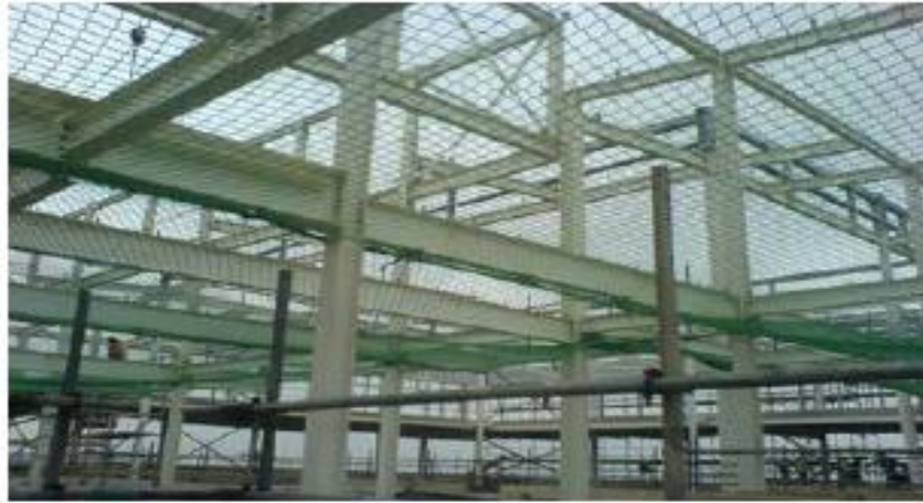
Safety net installed below the roof truss for height work
