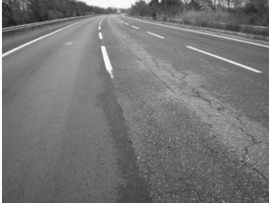
Figure 15.5 Reflective cracking initiated over an old paving joint in a flexible pavement.
