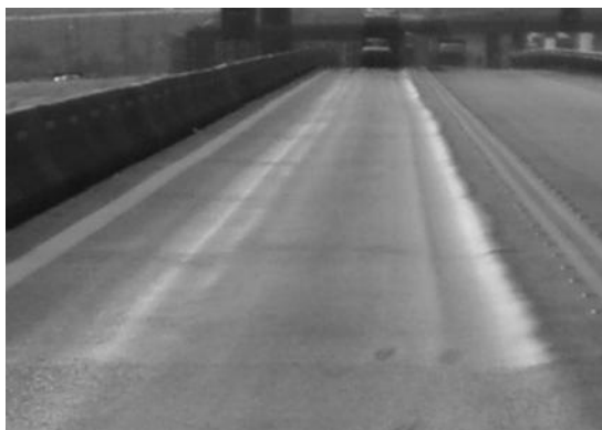
Figure 15.14 Typical rutting quite often formed very early, as shown schematically in Figure 15.12b.
