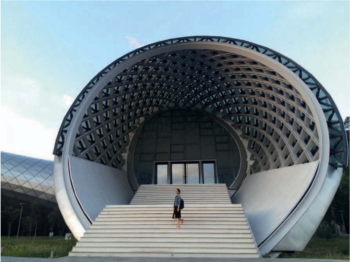
Figure 10.27 Entrance, Music Theatre and Exhibition Hall, Tbilisi, 2017; Massimiliano and Doriana Fuksas, architects. Although superficially similar to form-active grids (see Figure 10.5), forms like this are not directly related to structural function. The supporting steel frameworks are semi-form-active with relatively high levels of internal force requiring the use of substantial quantities of material to achieve adequate strength.
