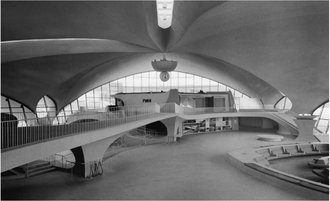
Figure 9.15a TWA Flight Centre, Idlewild (Kennedy) Airport, New York, 1962; Eero Saarinen, architect. The formalist free-form geometry of this building was related neither to structural function nor to simple mathematical description. The resulting semi-form-active structure generated large bending moments. The reinforced concrete envelope, which is often referred to erroneously as a 'thin shell', was problematic to construct and required large volumes of material to give it sufficient strength, in contrast to the lightweight shells designed by engineers such as Torroja and Candela. The building is no longer used for its original purpose and now serves as a 500-bedroom hotel.
