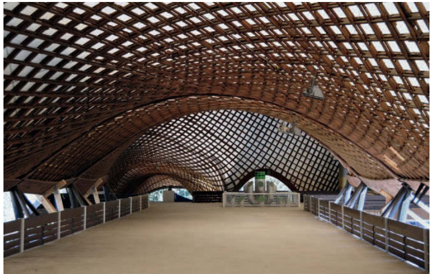
Figure 11.5 Multihalle, Bundesgartenschau, Mannheim, 1975; Carlfried Mutschler and Partners, architects; Ove Arup & Partners (Edmund (Ted) Happold), with Frei Otto, engineers. The 85 m principal span of this multi-space enclosure was achieved with a lightweight, form-active, timber grid-shell. An ingenious construction system was devised to allow the complex form to be built using straightforward techniques. The combination of sophistication and simplicity was similar to that found in the works of Nervi and Torroja.
