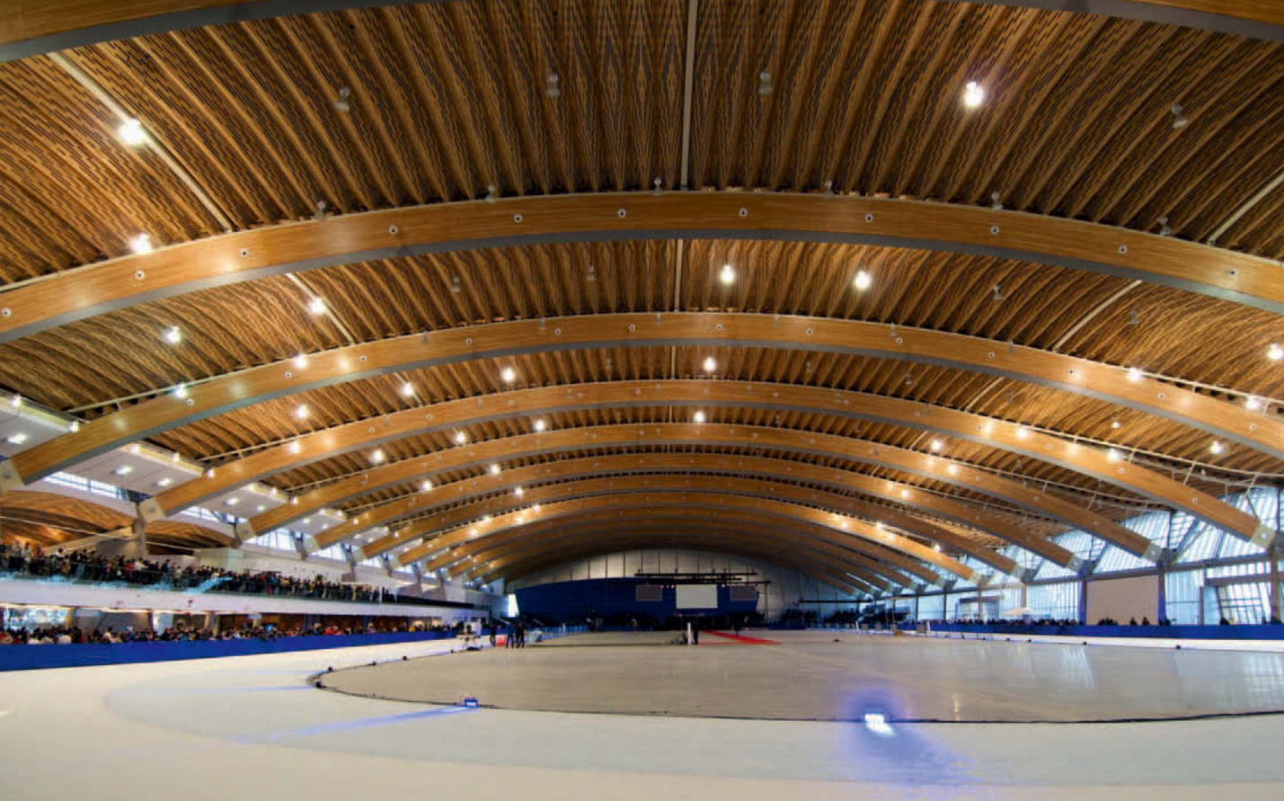
Figure 3.9 Olympic Oval, Richmond, Canada; CannonDesign, architects. The principal structural elements of this building, which received a LEED award for its many environmentally sustainable features, are composite arches of laminated timber and steel spanning 100 m.
