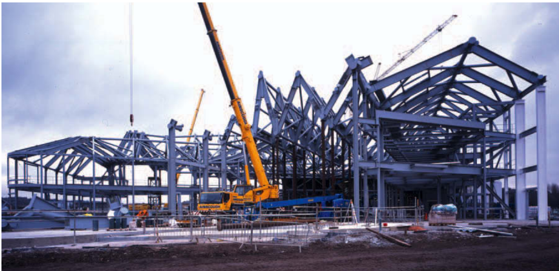
Figure 1.10 Riverside Museum, Glasgow, 2012; Zaha Hadid, architect; Buro Happold Engineering, engineers. Due to its unconventional structural configuration, a massively strong steel framework structure was required.
