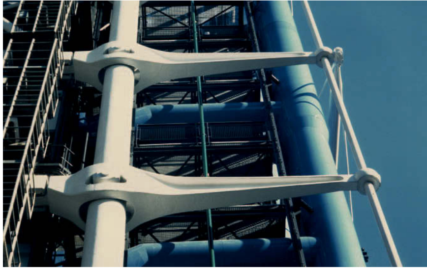
Figure 9.30 Gerberette brackets, Centre Pompidou, Paris, 1978; Piano and Rogers, architects; Ove Arup & Partners (Peter Rice), structural engineers. The floor girders are attached to the inner ends of these brackets, which pivot on hinge pins through the columns. The weights of the floors are counterbalanced by tie forces applied at the outer ends of the brackets. The arrangement sends 25% more force into the columns than would have occurred if the floor beams had been attached to them directly. Fabrication by casting allowed a very neat appearance and reintroduced the technique to architecture for the shaping of major components.
