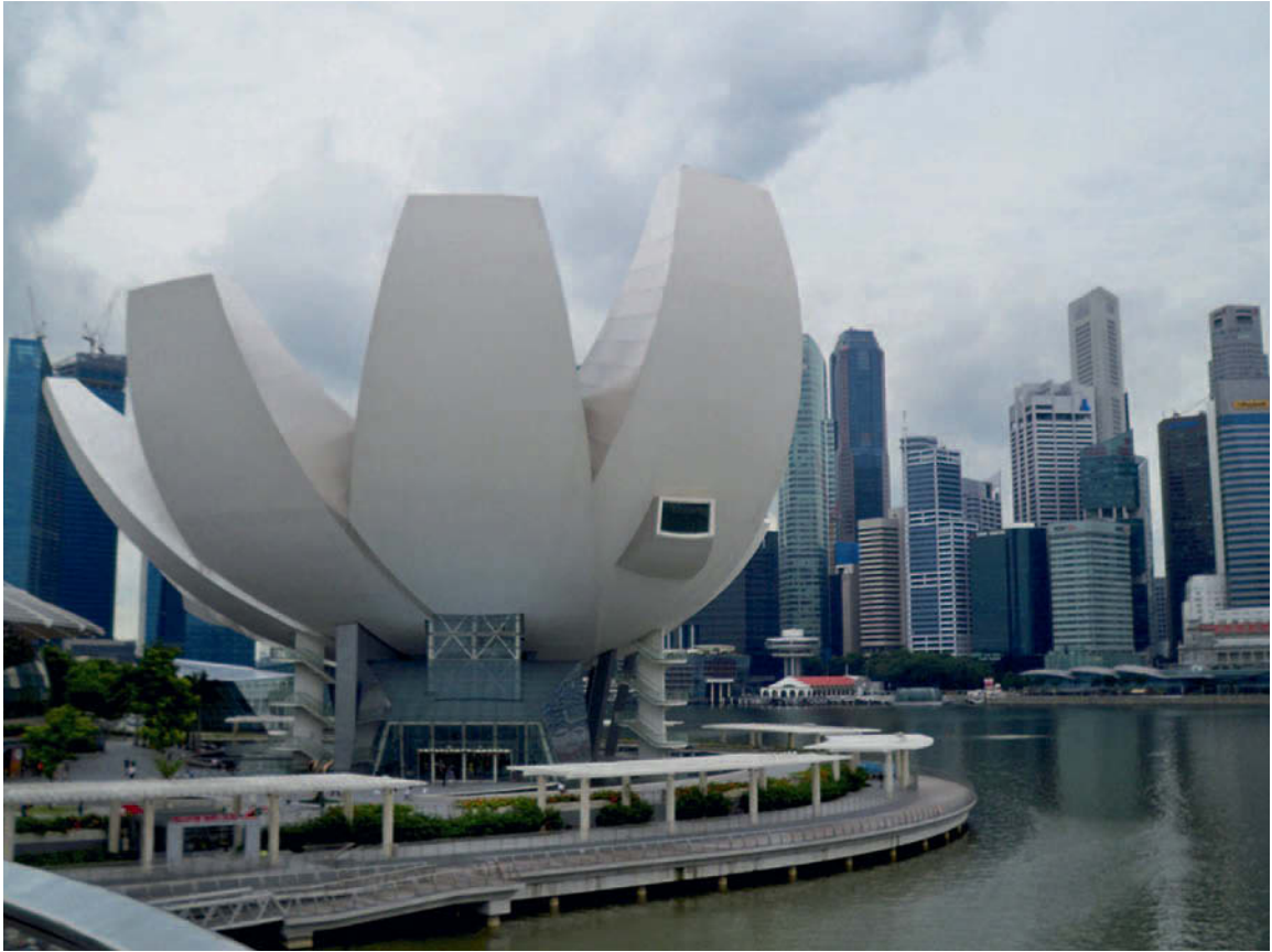
Figure 10.28 ArtScience Museum, Marina Bay Sands, Singapore, 2011; Moshe Safdie, architect; Arups, engineers. Complex forms such as this generate high internal forces, because they are unrelated to structural function, and are difficult to design and construct. In this case an elaborate steel lattice framework supports a skin of fibre-reinforced polymer. The fabric of the building performs poorly in respect of sustainability criteria.
