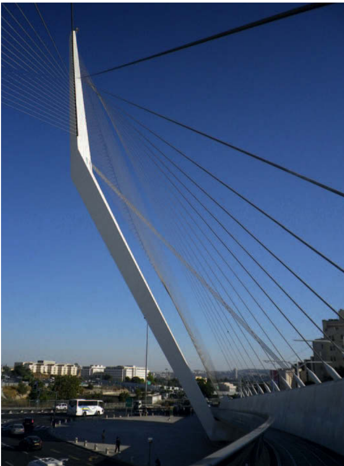
Figure 9.19 Chords bridge, Jerusalem, 2008; Santiago Calatrava, engineer. The out-of-balance forces caused by the eccentric position of the supporting mast of this cable-stayed bridge are compensated for by the horizontal-arch effect of the deck. The complex geometry produces a spectacular network of support cables, some of which are used directly to stabilise the mast.
