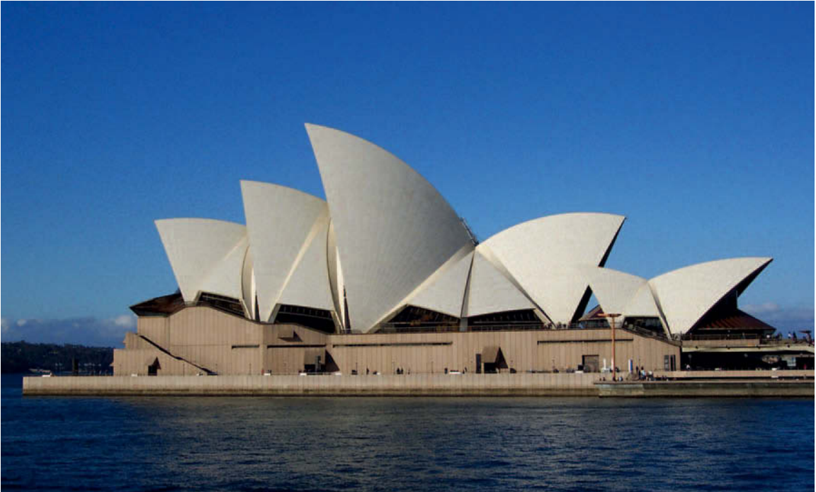
Figure 9.25 Sydney Opera House, Sydney, 1958–1972; Jørn Utzon, architect; Ove Arup & Partners, engineers. Although often referred to as ‘shells’ (which, in structural terms, they are not), the distinctive forms of this building were constructed as a series of linked semi-form-active portal frameworks clad in non-structural pre-cast concrete panels faced with ceramic tiles.
