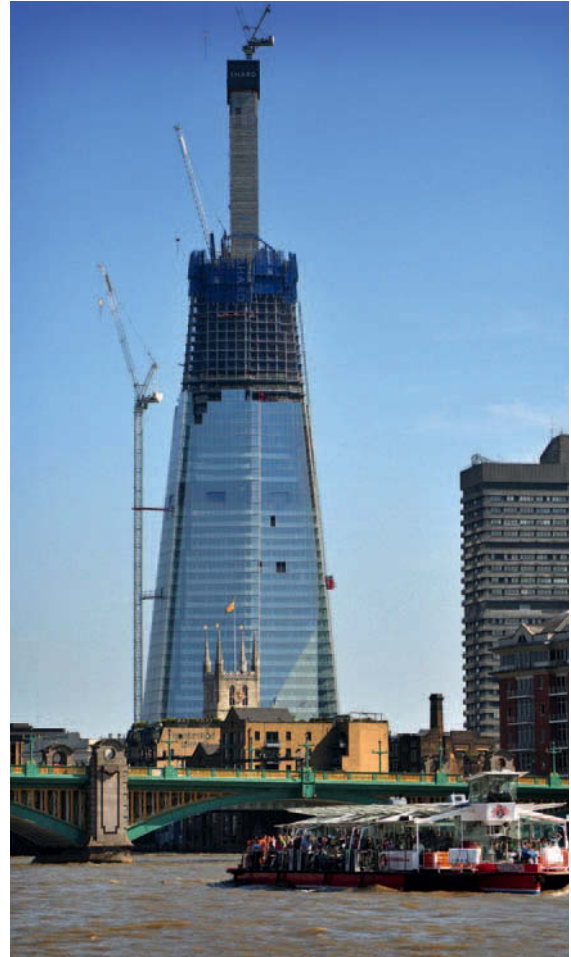
Figure 10.16b The Shard, London, 2013; Renzo Piano Building Workshop, architects; WSP Cantor Seinuk, engineers. The building has a composite steel and reinforced concrete structure with the concrete core (seen exposed in this progress shot) providing the principal resistance to lateral load. In addition to the normal considerations that affect the design of very tall buildings, the implication of the collapse of the World Trade Centre in 2001 influenced the structural design. As with many of the world's most recently completed very tall buildings, it is doubtful if The Shard should be considered as an example of structure as architecture because, apart from the tapering profile, structural requirements had little effect on its appearance. The current state of structural technology would in fact have allowed a non-tapering profile to be adopted so the taper could be considered to be a stylistic device.
