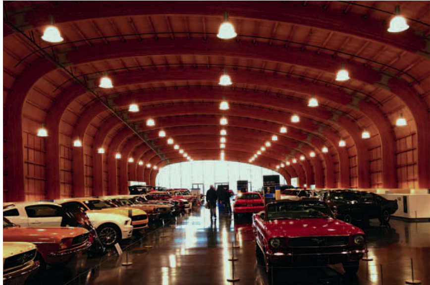
Figure 3.4 LeMay Museum, Tacoma, 2012; Large Architecture, architects. The principal structural elements here are laminated timber frameworks (1.3 m x 22 mm in cross-section) which span 32 m across the rectangular-plan interior.
