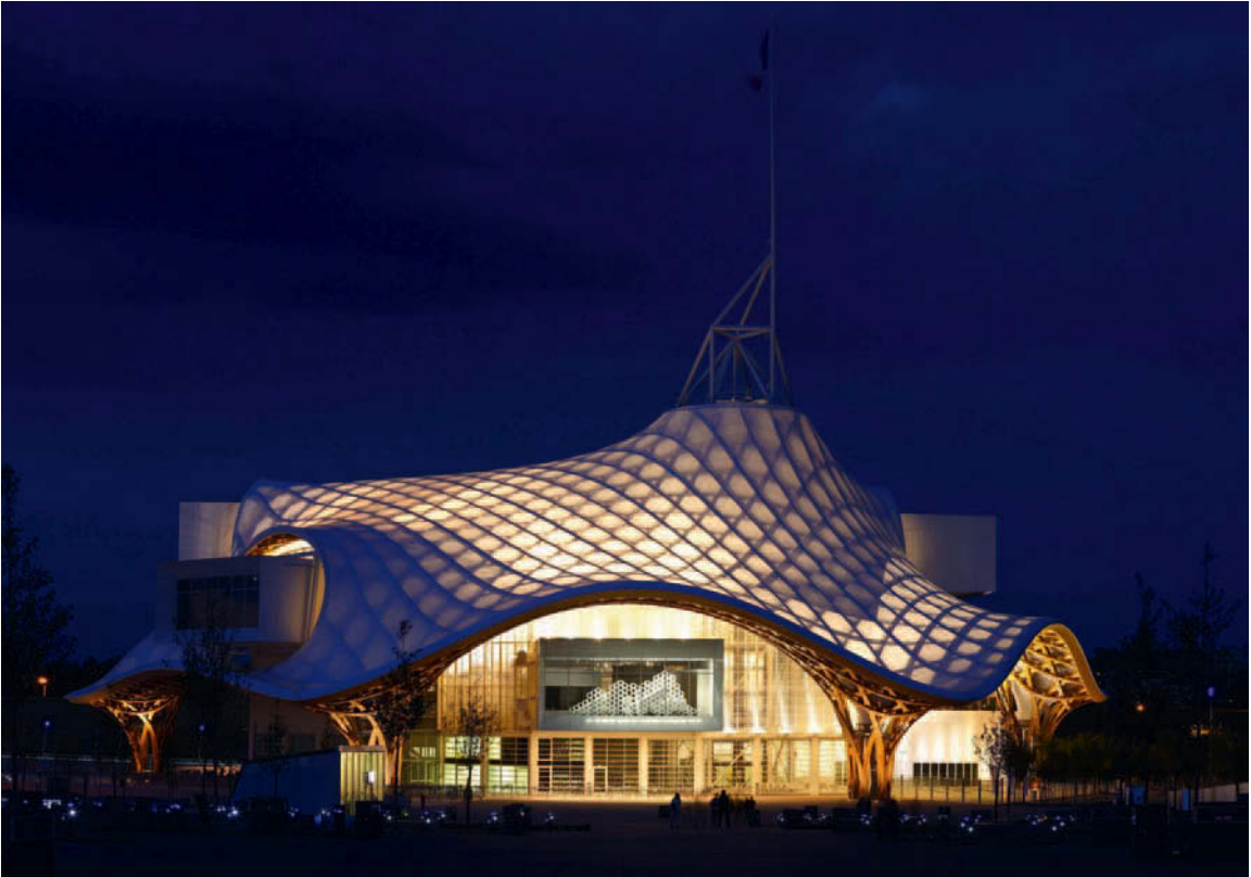
Figure 11.6 Centre Pompidou-Metz, France, 2010; Shigeru Ban, architect; Arups (Cecil Balmond), engineers. The 90 m-span roof canopy of this building is a timber lattice grid-shell of similar configuration to that at the Multihalle at Mannheim, designed with the aid of recent form-determining software. The building demonstrates the continuing feasibility of using timber for large-scale public buildings.
