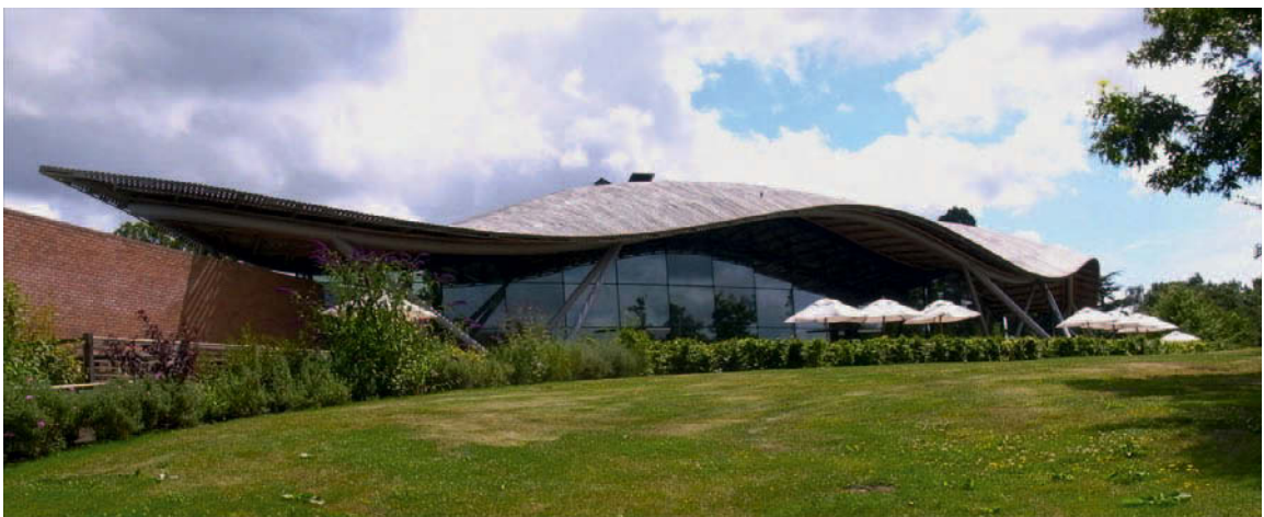
Figure 3.10 Savill Building, Windsor, UK, 2006; Glen Howells Architects, architects; Buro Happold Engineering and Haskins Robinson Waters, engineers. The primary structural element in this building is a timber grid-shell, spanning 90 x 25 m, constructed from locally sourced larch and oak.
