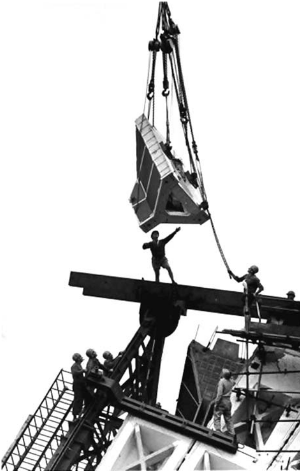
Figure 9.27 Sydney Opera House, Sydney, 1958–1972; Jørn Utzon, architect; Ove Arup & Partners, engineers. The frameworks at Sydney were constructed in pre-cast sections that were sufficiently small to be lifted by the largest cranes then available. The massive volumes of concrete required to provide sufficient strength contrast with the thin shells designed by engineers such as Torroja and Candela, which achieved much greater spans with concrete thicknesses of around 100 mm.
