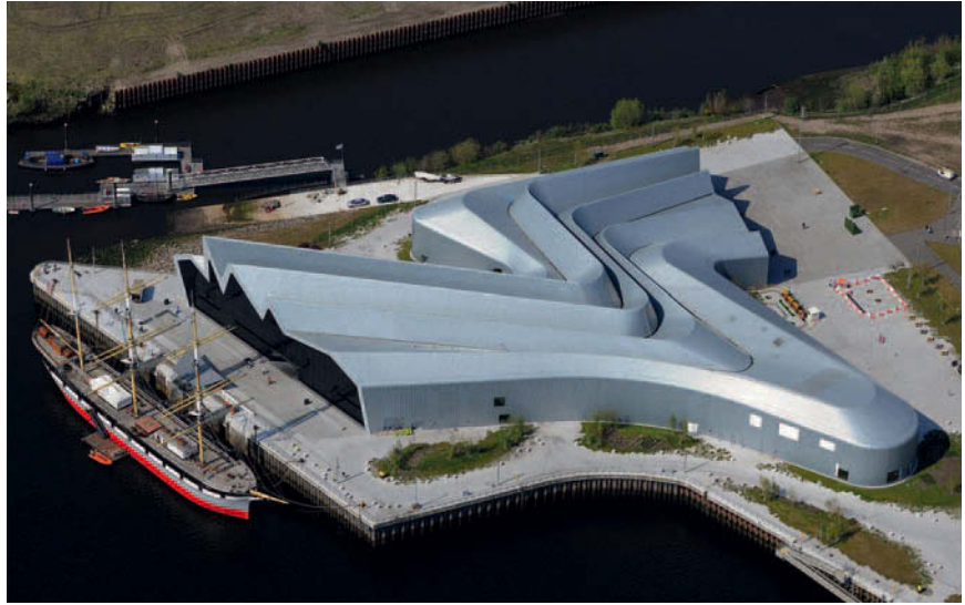
Figure 10.25 Riverside Museum, Glasgow, 2011; Zaha Hadid, architect, Buro Happold, Engineering, engineers. The Z-form plan of the building, together with the single-volume gallery space that runs its full length, are intended to allow the building to be a 'mediator between city and river'. The irregularly varying serrated cross-section can be seen as 'a cityscape and a responsive gesture to encapsulate waves on water'.
