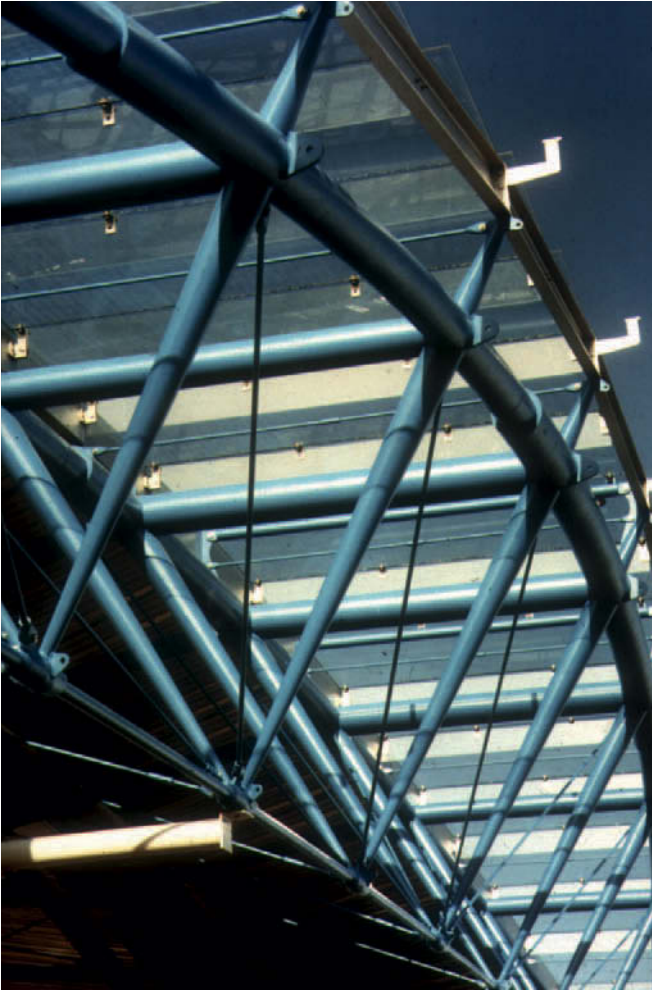
Figure 10.5 International Terminal, Waterloo Station, London, 1992; Nicolas Grimshaw, architect; Anthony Hunt Associates, engineers. The general arrangement of the principal trusses was determined from structural considerations. The compressive upper elements are larger than the single tensile tie rod so as to be capable of resisting buckling. The scantlings that connect the two sets of elements are tapered mainly for visual reasons. Photo: Anthony Hunt Associates.
