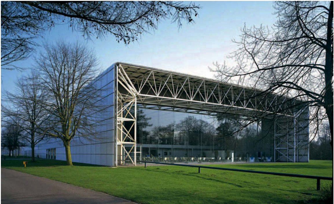
Figure 9.33 Sainsbury Centre for the Visual Arts, Norwich, 1978; Foster Associates, architects; Anthony Hunt Associates, engineers. With its clean-cut lines and simplicity of form this building exemplifies Foster's approach to architecture. The cross-sectional shape is far from ideal structurally, considering the relatively long span of 35 m, and many compromises with structural performance were required to provide adequate support for the bespoke cladding system. The internal environment of the thinly-clad single-volume enclosure proved to be highly problematic in respect of conservation of the art objects which it was intended to house and display. Appearance, rather than function, was the principal driver of the design.
