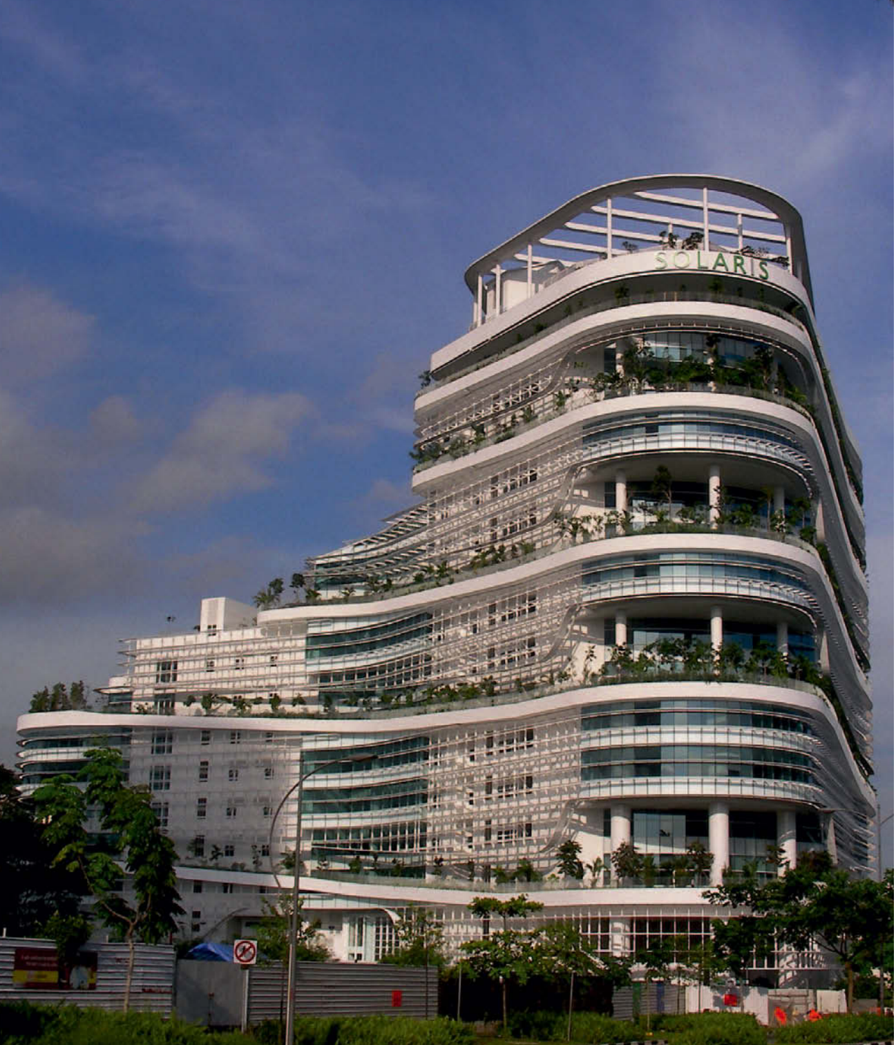
Figure 1.7 Solaris Building, Singapore, 2011; T. R. Hamzah & Yeang, architects; Arups, engineers. Ecological and sustainability considerations greatly influenced the design of this building. The structural armature is a reinforced concrete framework that allowed the creation of irregular plan-forms and facilitated the inclusion of green corridors and a passively ventilated atrium.
