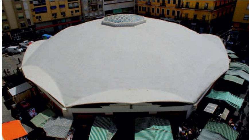
Figure 9.7 Algeciras market hall, 1934; Eduardo Torroja, engineer; Manuel Arcas, architect. Using a spherical approximation to the form-active shape, a span of 47.7 m was achieved with a maximum shell thickness of 100 mm. The shell is stiffened by cylindrical mini-canopies at its perimeter. Outward thrusts are absorbed by a tie beam at the tops of the supporting columns.
