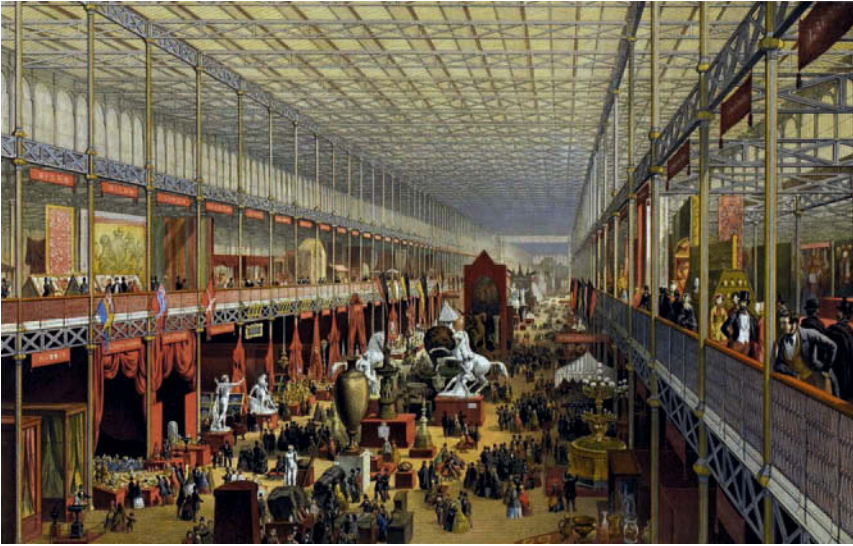
Figure 8.5 The Crystal Palace, London, 1851; Joseph Paxton, designer. The building performs well as a structure. The non-form-active, post-and-beam typology, with ‘improved’ triangulated horizontal elements, is entirely appropriate for the spans involved.
