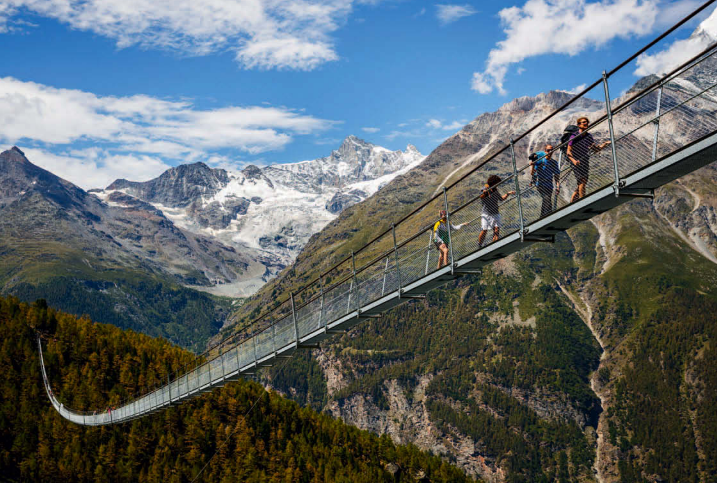
Figure 4.6 The Charles Kuonen Suspension Bridge, Randa, Switzerland, 2017; Swissrope, constructor. The steel ropes that support the footway are form-active structures and demonstrate the very high structural efficiency that this typology makes possible.
