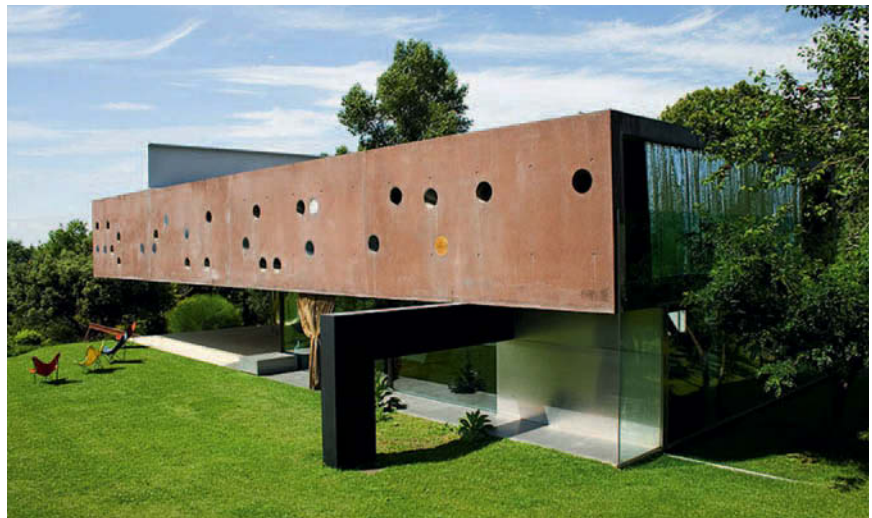
Figure 9.37 Maison de Floirac, Bordeaux, France, 1998; Rem Koolhaas OMA, architects; Arups (Cecil Balmond), engineers. The architectural concept was of a box up in the air (containing bedrooms) floating on a glass-walled living space which could open out to the landscape and vanish. Considerable ingenuity was required to realise the structure. The box was formed by a chequerboard of intersecting reinforced concrete walls and was supported on two offset steel frameworks (both partially visible). The degree of collaboration between architect and engineer was significant.
