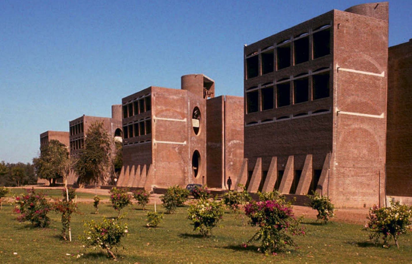
Figure 5.6 Indian Institute of Management, Ahmedabad, India, 1974; Louis Kahn and Balkrishna Vithaldas Doshi, architects. Extensive use was made of loadbearing masonry in the structure of this building complex, which contains both multi-cellular and large single-cell interior spaces. Horizontal structures are of reinforced concrete.
