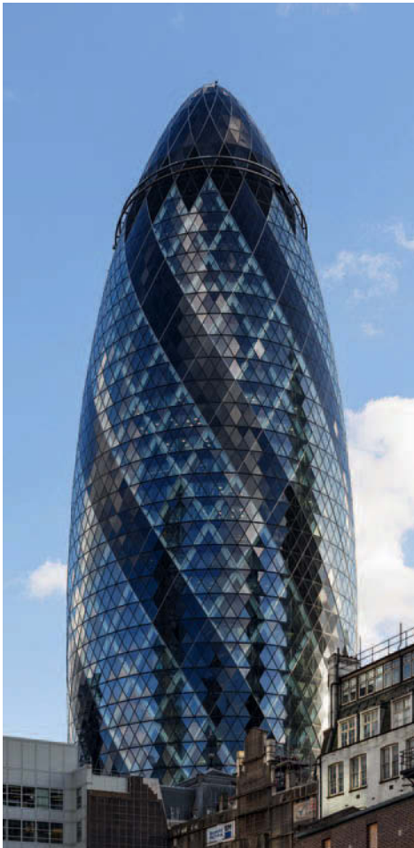
Figure 11.1 30 St Mary Axe ('The Gherkin'), London, 2004; Foster & Partners, architects; Arups, engineers. 'London's first ecological tall building', was the claim made by the architects; this may well be legitimate in view of the 'green' features that were incorporated.
