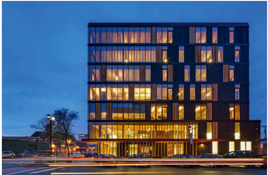
Figure 11.11 Wood Innovation and Design Centre building, Prince George, British Columbia, Canada, 2014; Michael Green Architecture, architects; Equilibrium Consulting, engineers. The structure of this multi-storey academic and laboratory building is entirely of timber.
