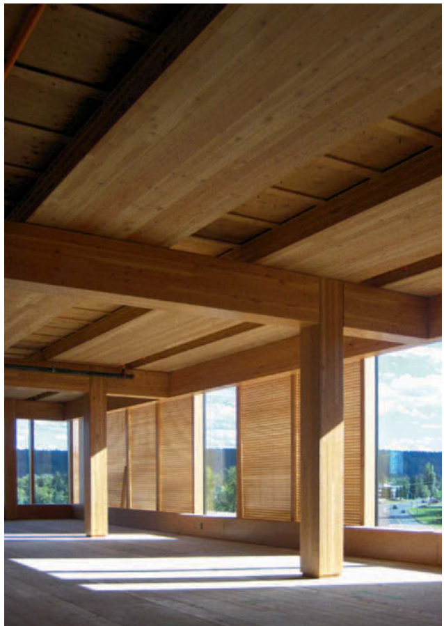
Figure 11.12 Wood Innovation and Design Centre building, Prince George, British Columbia, Canada, 2014; Michael Green Architecture, architects; Equilibrium Consulting, engineers. The beams and columns of the building are of laminated timber. The floor decks are also constructed entirely of timber.
