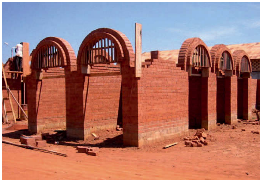
Figure 11.14 Central Market complex, Koudougou, Burkina Faso, 1999–2005; Swiss Agency for Development and Cooperation, architects and project directors. Design for low environmental impact involves the adoption of forms that are structurally efficient, so as to minimise the use of material, and that are appropriate for their constituent materials. This is a context in which a purely formalist approach to architectural design is unlikely to be successful.
