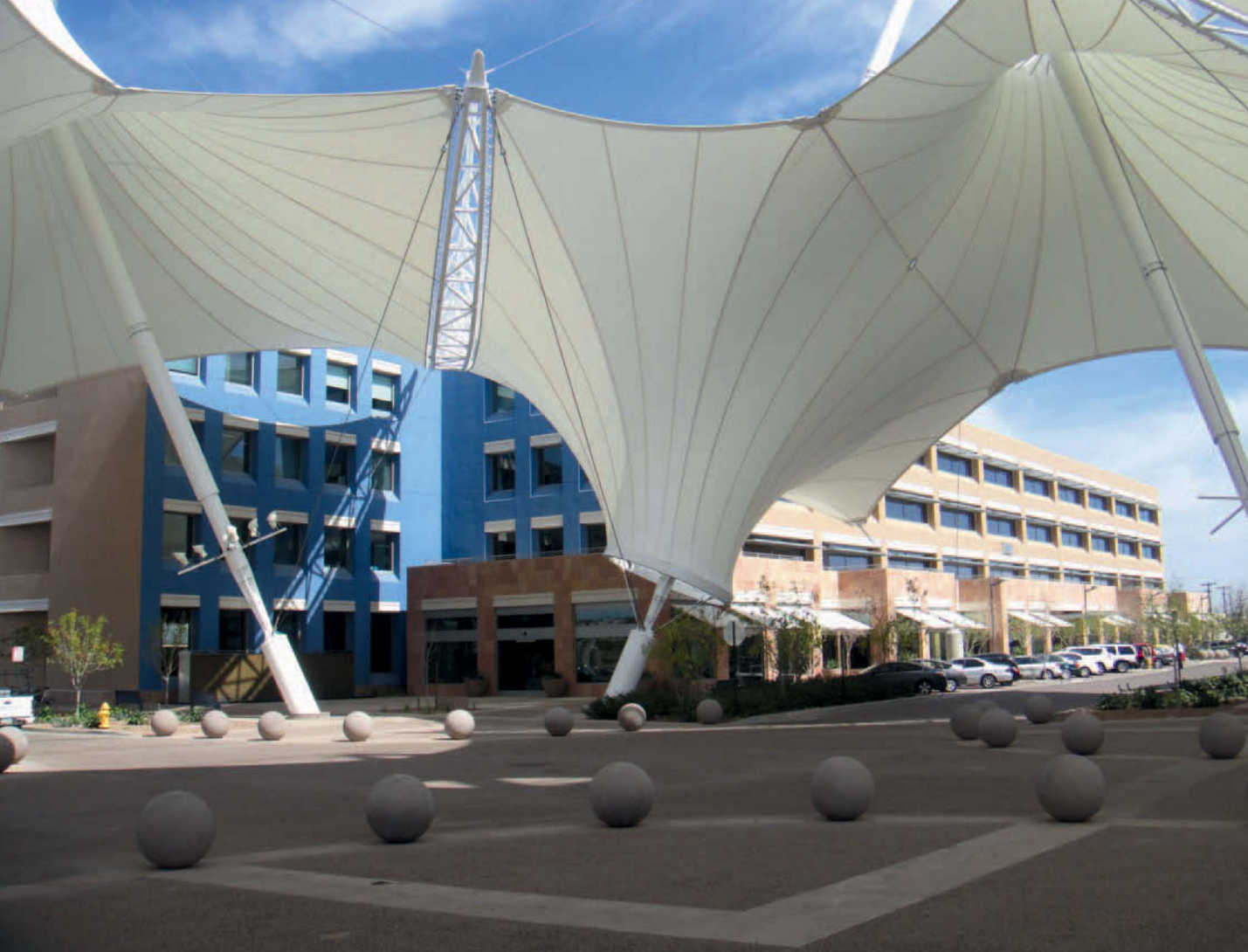
Figure 5.19 SkySong: ASU Scottsdale Innovation Centre, Arizona, USA, 2009; FTL Design Engineering Studio, architects. The canopy of this structure is a tensile membrane with a form-active geometry. Although flexible structures will always adopt the form-active shape for the load involved, thus restricting the choices of the designer, variations in form can be produced by manipulating the boundary (support) conditions, as here.
