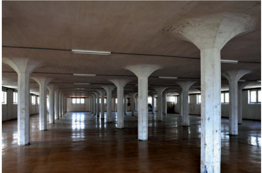
Figure 8.9 Flat-slab structure, Grain Depot, Altdorf, 1912; Robert Maillart, engineer. The flat-slab system, now one of the commonest forms of multi-storey structure, was developed by Robert Maillart. In its most economic form it is based on a regular square column grid but its two-way spanning capability can allow the slabs to be supported on an irregular basis. It was the planning freedom and sculptural possibilities that this enables that attracted the attention of Giedion.
