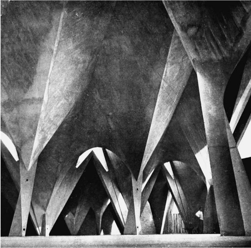
Figure 9.14 Church of Our Lady of the Miraculous Medal, Mexico City, 1955; Felix Candela, architect/engineer. A highly architectural use of the hyperbolic paraboloid geometry.
