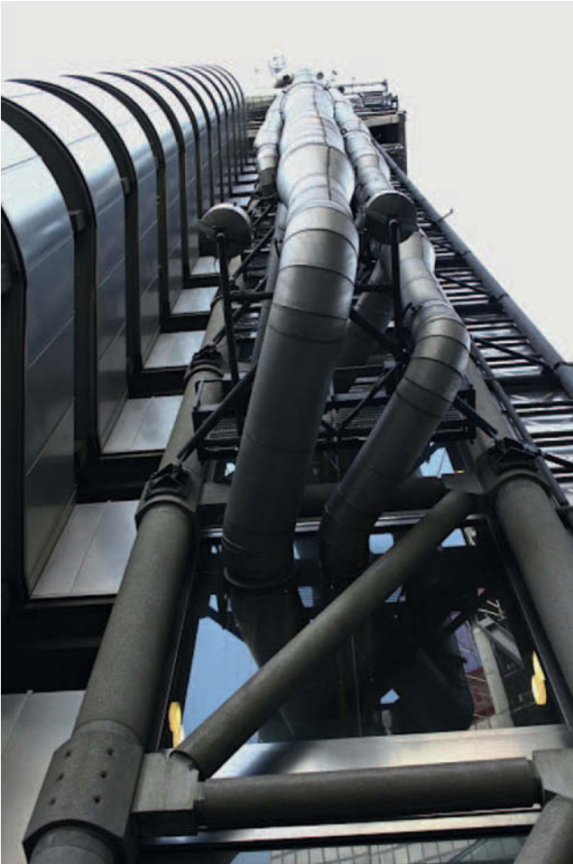
Figure 10.9 Lloyd's headquarters building, London, 1986; Richard Rogers & Partners, architects; Ove Arup & Partners, engineers. Ducts and other services hardware are exposed on the exterior of the building.
