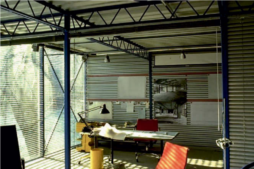
Figure 6.5 Hopkins House, London, UK, 1977; Michael and Patty Hopkins, architects; Anthony Hunt Associates, structural engineers. The very short spans involved here would not normally justify the use of complex triangulated elements for the horizontal structure. Ease and speed of erection were the main technical reasons for their selection. The visual interest that they produce was nevertheless the principal reason for their adoption.
