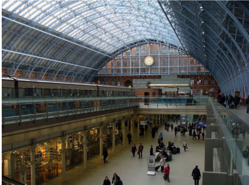
Figure 9.1 Train shed, St Pancras Station, London, 1868; William Henry Barlow and Rowland Mason Ordish, engineers. The clear span across the entire width of the platforms was justified here by operational requirements. At 73 m it was the largest in the world when constructed. The use of a form-active parabolic arch profile was appropriate as was the 'improvement' by triangulation of the principal structural elements. The resulting striking architectural space was generated from the satisfaction of purely functional requirements.
