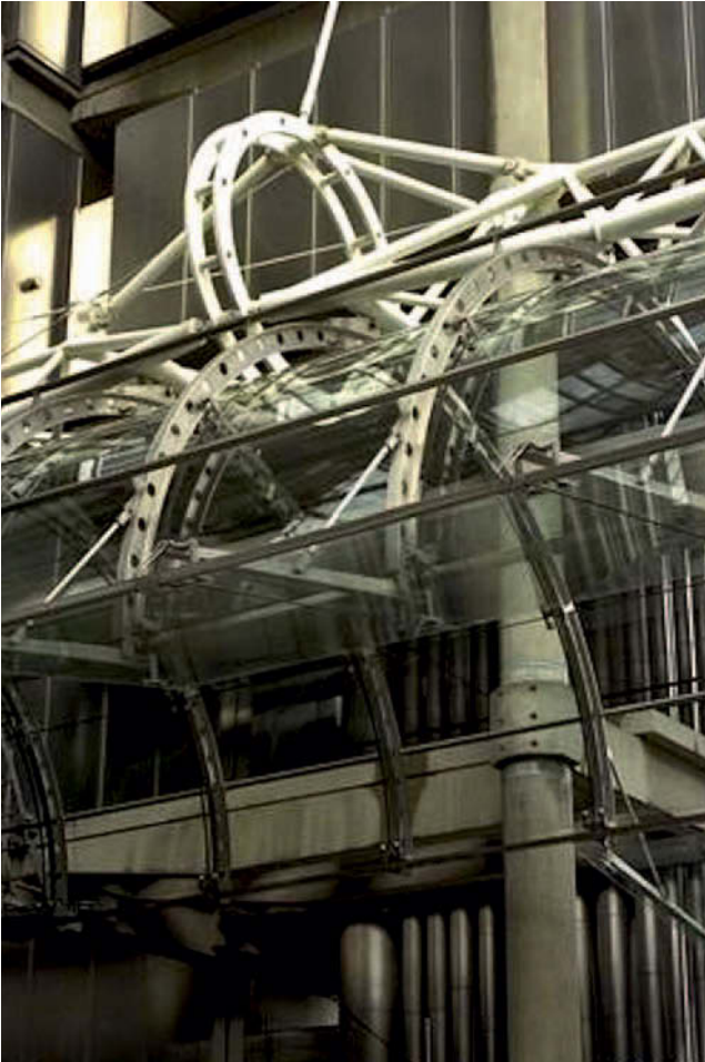
Figure 10.6 Entrance canopy, Lloyd's headquarters building, London, 1986; Richard Rogers & Partners, architects; Ove Arup & Partners, engineers. The curved steel ribs with circular 'lightening' holes are reminiscent of structures found in the aerospace industry.
