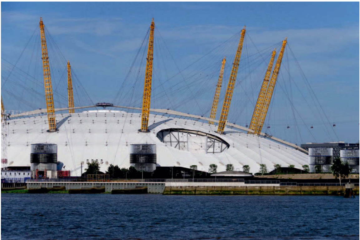
Figure 10.13 Millennium Dome, London, 1999; Richard Rogers & Partners, architects; Buro Happold Engineering, engineers. This is a mast-supported, dome-shaped cable network with a diameter of 358 m (span c. 225 m). The use of a tensile form-active structure is fully justified for spans of this size and determines the overall form of the building.
