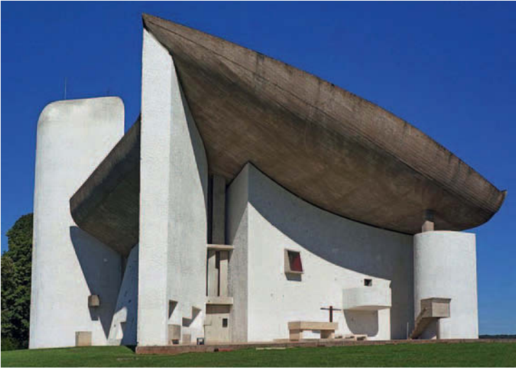
Figure 10.22 Chapel of Notre-Dame du Haut, Ronchamp, France, 1954; Le Corbusier, architect. Structural considerations played very little part in the determination of the form of this building. Its small scale together with the excellent structural properties of reinforced concrete, which was used for the roof, meant that it could be constructed without difficulty.
