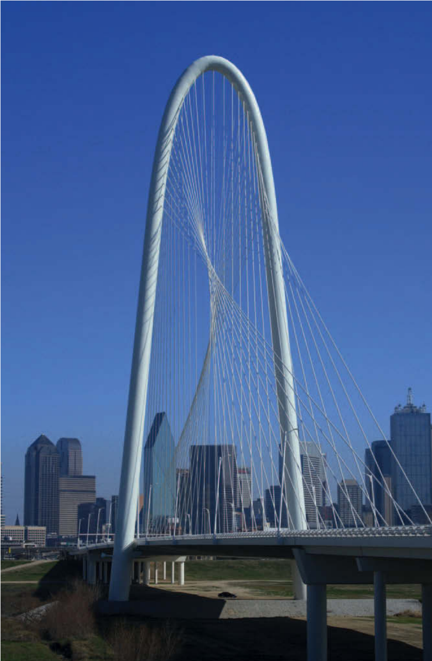
Figure 9.20 Margaret Hunt Hill bridge, Dallas, 2012; Santiago Calatrava, engineer. The device that produced the spectacular network of cables in this bridge was the use of a transverse arch rather than a mast as the vertical structural element. The cables are splayed from the crown of the arch to a single, central spine beam in the deck. The avoidance of eccentricity, as the creator of visual interest, resulted in a more satisfactory structural performance than was achieved with either of the other two examples of bridges by Calatrava shown here.
