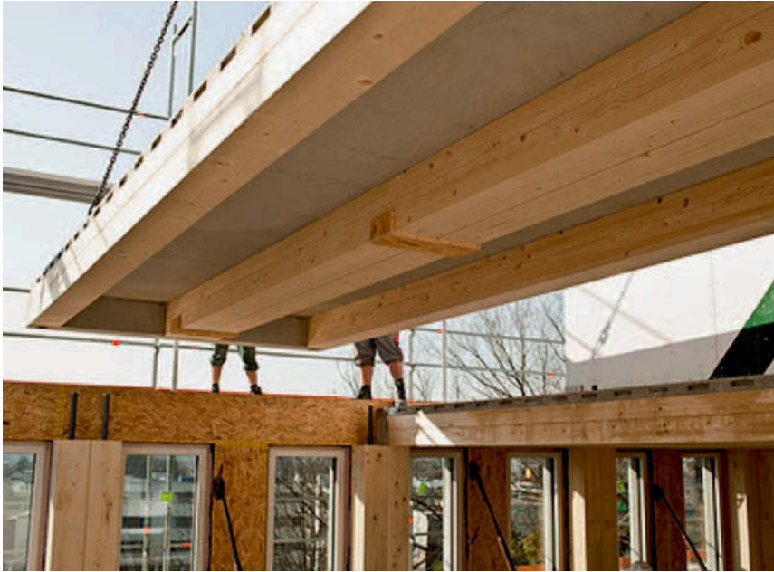
Figure 11.10 LifeCycle Tower One (LCT ONE), Dornbirn, 2013; Hermann Kaufmann, architect. Composite timber/pre-cast concrete floor slab units are supported on closely spaced timber columns. Most of the major components may be easily recycled.
