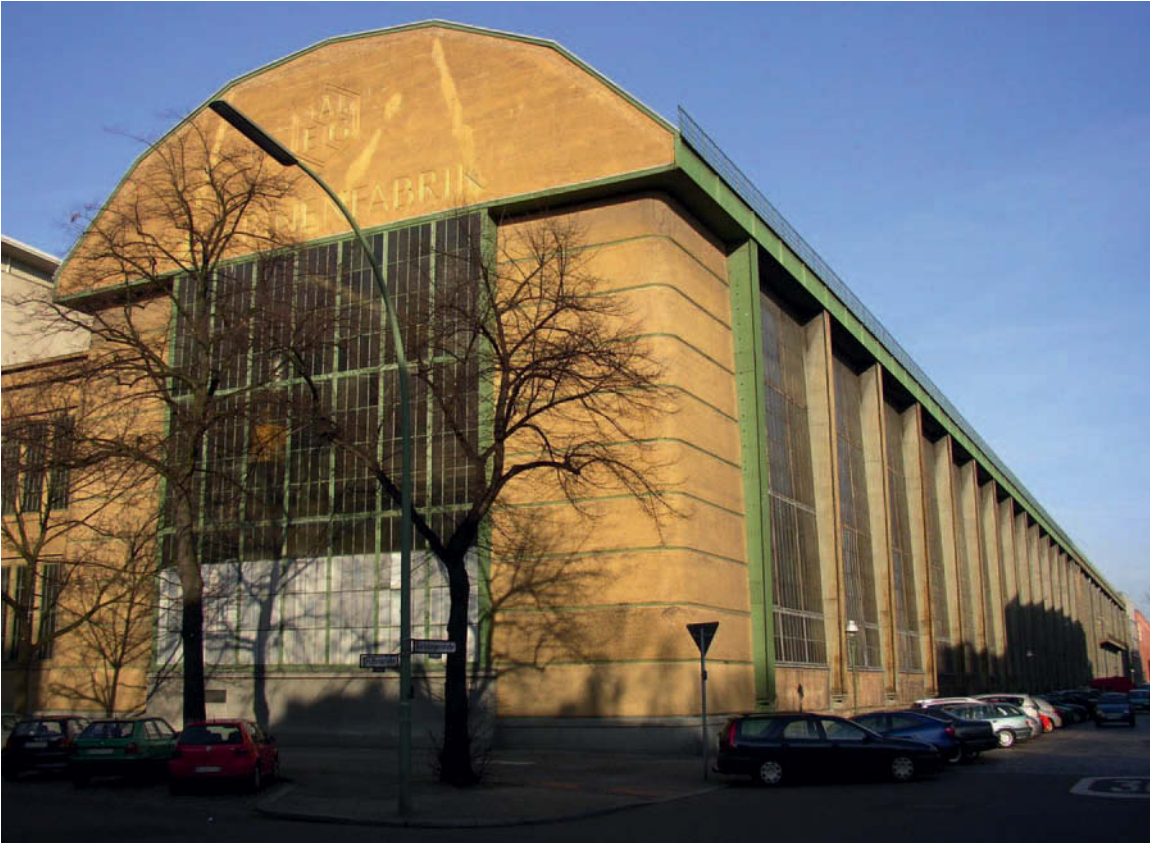
Figure 10.3 AEG Turbine Hall, Berlin, 1908; Peter Behrens, architect. Glass and structure alternate on the side walls of this building and the rhythm of the steel structure, which is exposed on the exterior, forms a significant component of the visual vocabulary. Unlike in many later buildings of the Modern Movement the structure was used 'honestly'; it was modified slightly for purely visual effect, but not to the detriment of its function.
