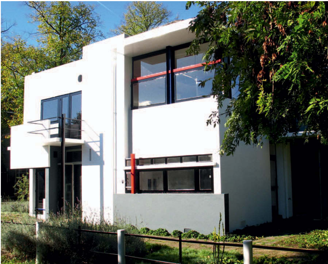
Figure 8.12 Schröder House, Utrecht, 1924; Gerrit Rietveld, architect. Although apparently suitable for realisation in slab-form concrete, this building is in fact a composite construction of brick masonry, timber and steel, with only minimal use of reinforced concrete slabs for the external balconies. A clever constructor can always find a way of making a building of this small size, without the need for the recourse to sophisticated reinforced concrete typologies implied by Giedion's advocacy of a necessary connection between avant-garde design and cutting-edge technology (see main text).
