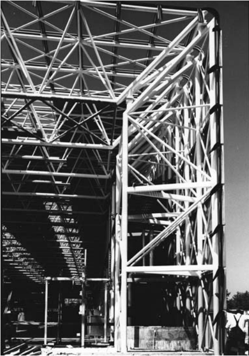
Figure 9.34 Sainsbury Centre for the Visual Arts, Norwich, 1978; Foster Associates, architects; Anthony Hunt Associates, engineers. This progress shot shows the bespoke cladding attached directly to the primary structural elements. A secondary structure of purlins and cladding rails, which would have allowed the primary elements to be more widely spaced with significant saving in material, was not possible due to the sensitivity of the cladding to movement. The cladding system failed and had to be replaced soon after the completion of the building for reasons unconnected to structural action.
