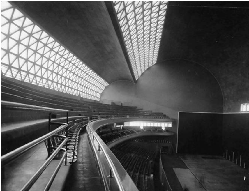
Figure 9.8 Frontón Recoletos, Madrid, 1935; Eduardo Torroja, engineer; Secundino Zuazo, architect. The roof of this building spans 55 m longitudinally between the end walls in an 'improved' beam configuration similar to that used by Nervi for the Orvieto Hangars. The shell thickness was 80 mm. Use of a simple cylindrical configuration resulted in a relatively simple construction process. A more complex profile, such as that used by Nervi with the Orvieto hangars, would not have been justified in this case.
