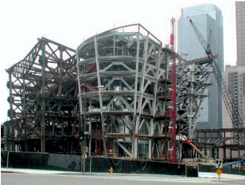
Figure 0.2 Walt Disney Concert Hall, Los Angeles; Frank Gehry (1929– ), architect. The supporting structural steel framework is highly inefficient. The overall cost of the building was $274 million, compared to $190 (equivalent) for three other halls on the same site that were built in the 1960s with conventional post-and-beam structures.
