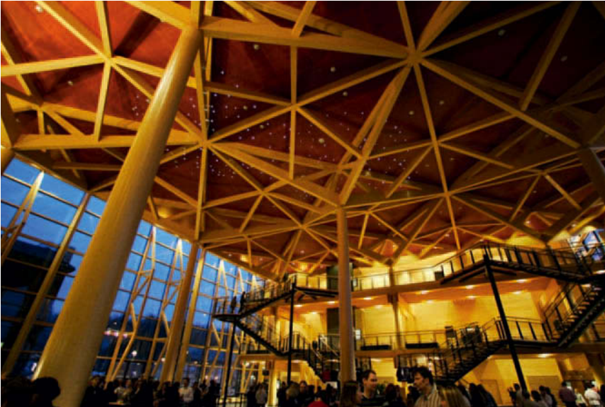
Figure 11.8 Sibelius Hall, Lahti, 2000; Kimmo Lintula and Hannu Tikka, architects; Turun Juva Oy, engineers. The structure of this large building, which includes a 1,100-seat concert hall and an extensive foyer, is entirely of timber and includes laminated timber beams, triangulated trusses and composite, solid-timber and plywood stressed-skin elements. The building demonstrates the continuing feasibility of timber structures for large-scale projects.
