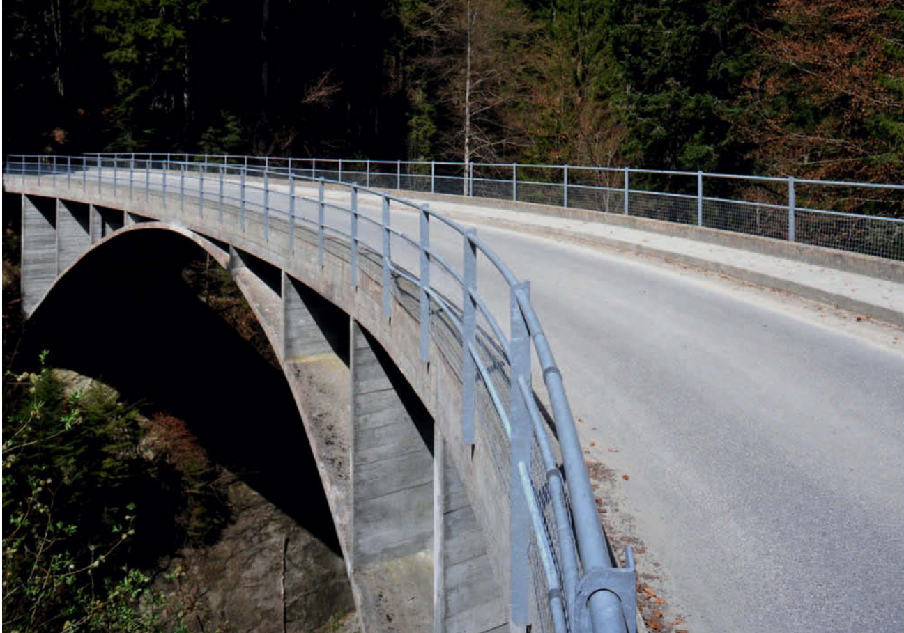
Figure 8.8 Schwandbach Bridge, Berne, 1933; Robert Maillart, engineer. The principal structural element of the bridge is a 37 m span, 200 mm thick, polygonal slab-form arch that supports the deck via 160 mm thick cross-walls. The polygonal profile of the slender arch, which is stiffened against buckling by the deck slab, is form-active in response to the concentrated loads transmitted by the cross-walls. In its form and simplicity the structure is entirely functional and devoid of ornamentation. For Giedion, it was a prime example of functional design but the transfer of the underlying design methodology to architecture was problematic, mainly because it lacked a cultural dimension, something that was not acknowledged by Giedion.
