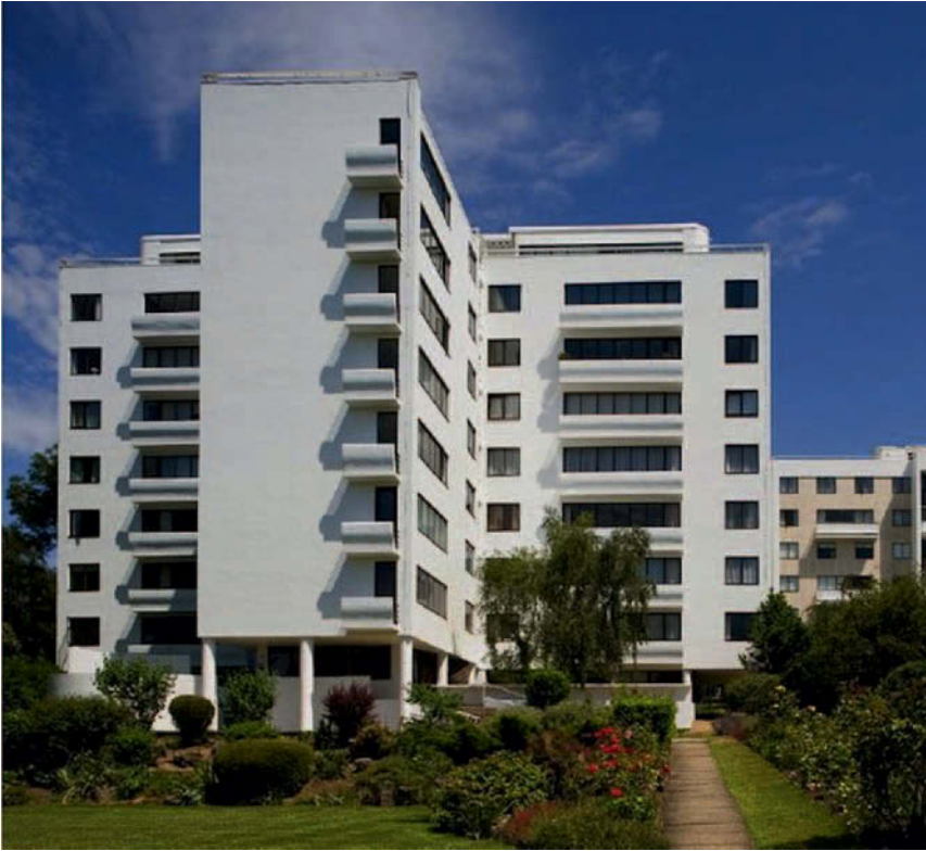
Figure 9.22 Highpoint I, London, UK, 1935; Berthold Lubetkin, architect; Ove Arup, structural engineer. The structure of this building is of reinforced concrete slabs in both vertical and horizontal planes. The non-form-active structural arrangement with solid slab cross-sections is entirely appropriate for the spans involved. The integration of architectural and engineering design considerations is remarkable and the result of close collaboration between architect and engineer through all stages of the design and construction.
