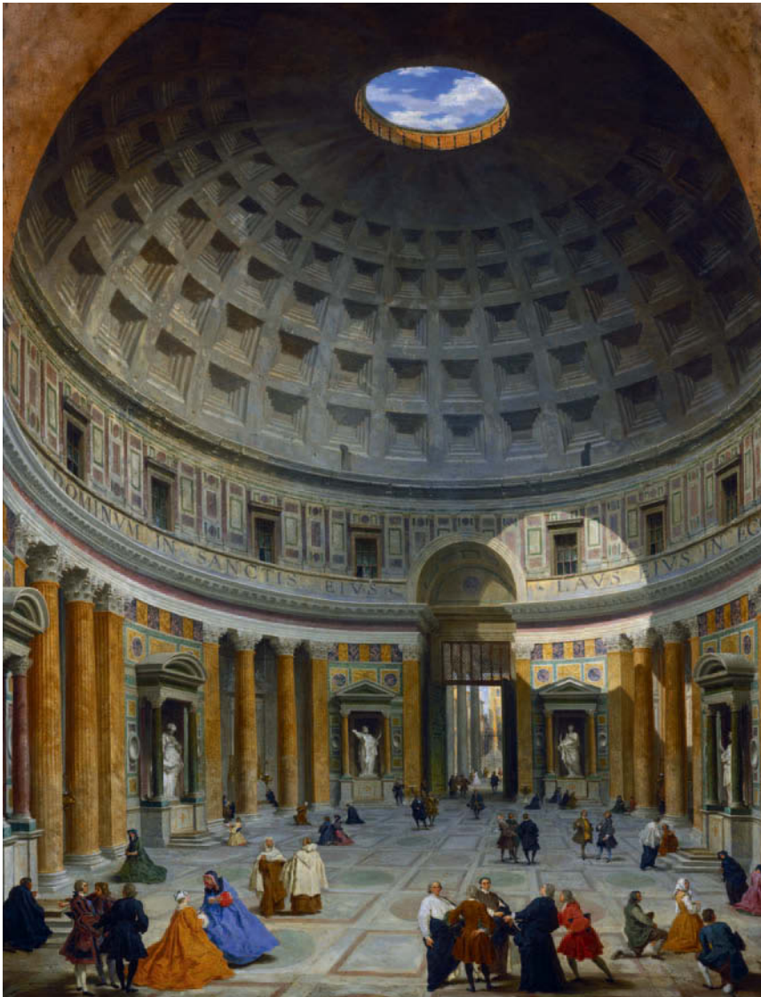
Figure 10.18 The Pantheon, Rome, C2 CE. The hemispherical concrete dome is supported on a cylindrical drum also of concrete. Both have thick cross-sections that have been 'improved' by the use of coffers or voids of various types and these technical devices have been incorporated into the visual scheme of the interior.
