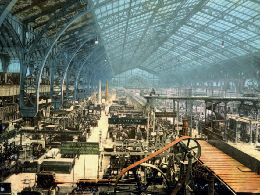
Figure 8.7 Galerie des Machines, Paris Exposition, 1889; Ferdinand Dutert, architect; Victor Contamin, engineer. The principal structural element of this building was a 115 m-span, three-hinge, triangulated steel portal framework. The use of an 'improved' semi-form-active structure was entirely justified for the span involved. Giedion correctly identified that the structural typology was distinctly different from the post-and-beam arrangement used for the smaller spans at the Crystal Palace. His conclusion that with this structure 'iron vaulting has found its true form' and had 'obliterated the division between load and support' is a poetic interpretation that adds drama to the pragmatism of the engineering.
