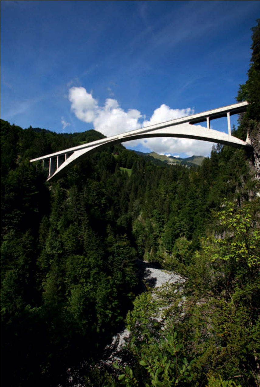
Figure 6.8 Salginatobel Bridge, Schiers, Switzerland, 1930; Robert Maillart, engineer.
