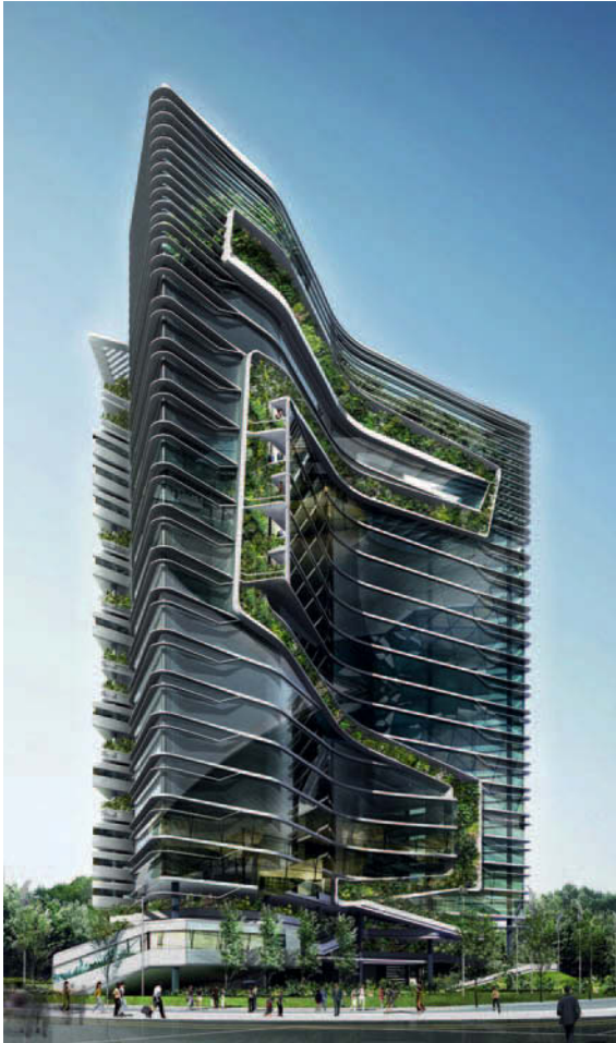
Figure 11.3 Spire Edge building, Manesar, India, 2013; T. R. Hamzah & Yeang Sdn Bhd, architects. Many 'sustainable' features were incorporated into this building, including a ramp-based 'green' corridor that ascends through every floor, a water harvesting, re-use and recycling system, and passive systems for lighting and ventilation. The green credentials of the building have inevitably been questioned, but it is nevertheless a rare example of a comprehensive approach being taken to address the problems that are posed by the design of large urban buildings that meet the criteria for sustainability. It is one of several examples by the architect Ken Yeang, a leading practitioner in the sustainability field.
