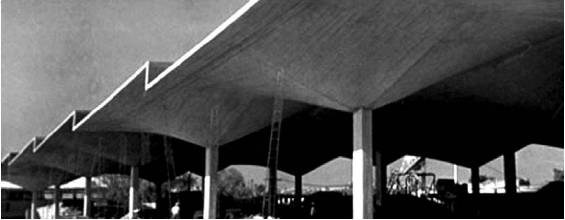
Figure 9.13 Umbrella hyper roof canopy, Mexico City, 1955; Felix Candela, engineer. Straight-sided elements of hyperbolic paraboloid shells are combined here to make a highly efficient roof canopy.
