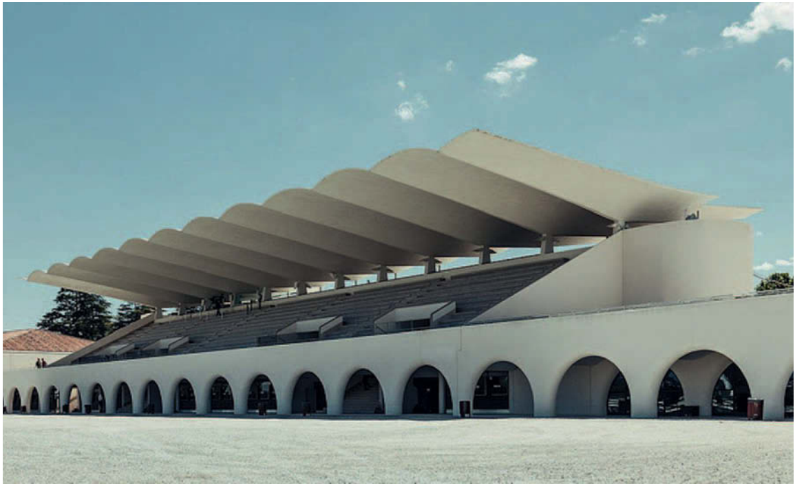
Figure 9.10 Zarzuela Hippodrome (racecourse) Pavilion, Madrid, 1935, Eduardo Torroja, engineer; Martín Domínguez Esteban and Carlos Arniches, architects. The oversailing reinforced concrete canopies are non-form-active cantilevers that have been given 'improved' cross-sections in the form of curved thin shells, greatly increasing their structural efficiency.
