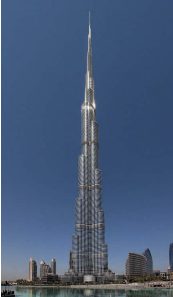
Figure 10.16a Burj Khalifa Building, Dubai, UAE, 2010; Skidmore, Owings & Merrill, architects and structural engineers. Multiple strategies were adopted in the structural design of this 'megatall' building, in which the principal structural material is reinforced concrete. The Y-shaped plan allowed the creation of shear walls in the wings to buttress the central hexagonal core. The tapering profile conformed to the intensity of bending produced by wind loading, which was minimised by aspects of the building's overall form. Technical consideration significantly influenced the appearance of the building.
