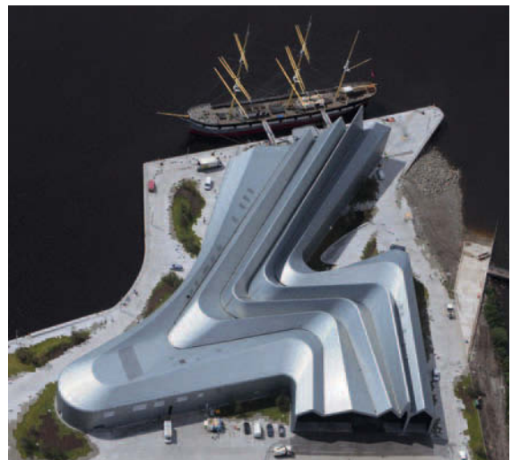
Figure 1.9 Riverside Museum, Glasgow, 2012; Zaha Hadid, architect; Buro Happold Engineering, engineers. The principal space in this building is an S-plan single exhibition area, of serrated cross-section, that runs through its entire length. The supporting structure is a steel skeleton framework that supports non-structural cladding. The glazed end of the building illustrates its cross-sectional shape.
