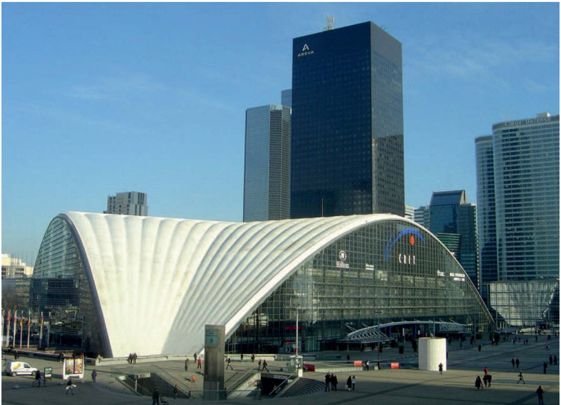
Figure 1.4 Exhibition Hall of the CNIT, Paris, 1958; Nicolas Esquillan, engineer. The principal element is a self-supporting reinforced concrete shell.
