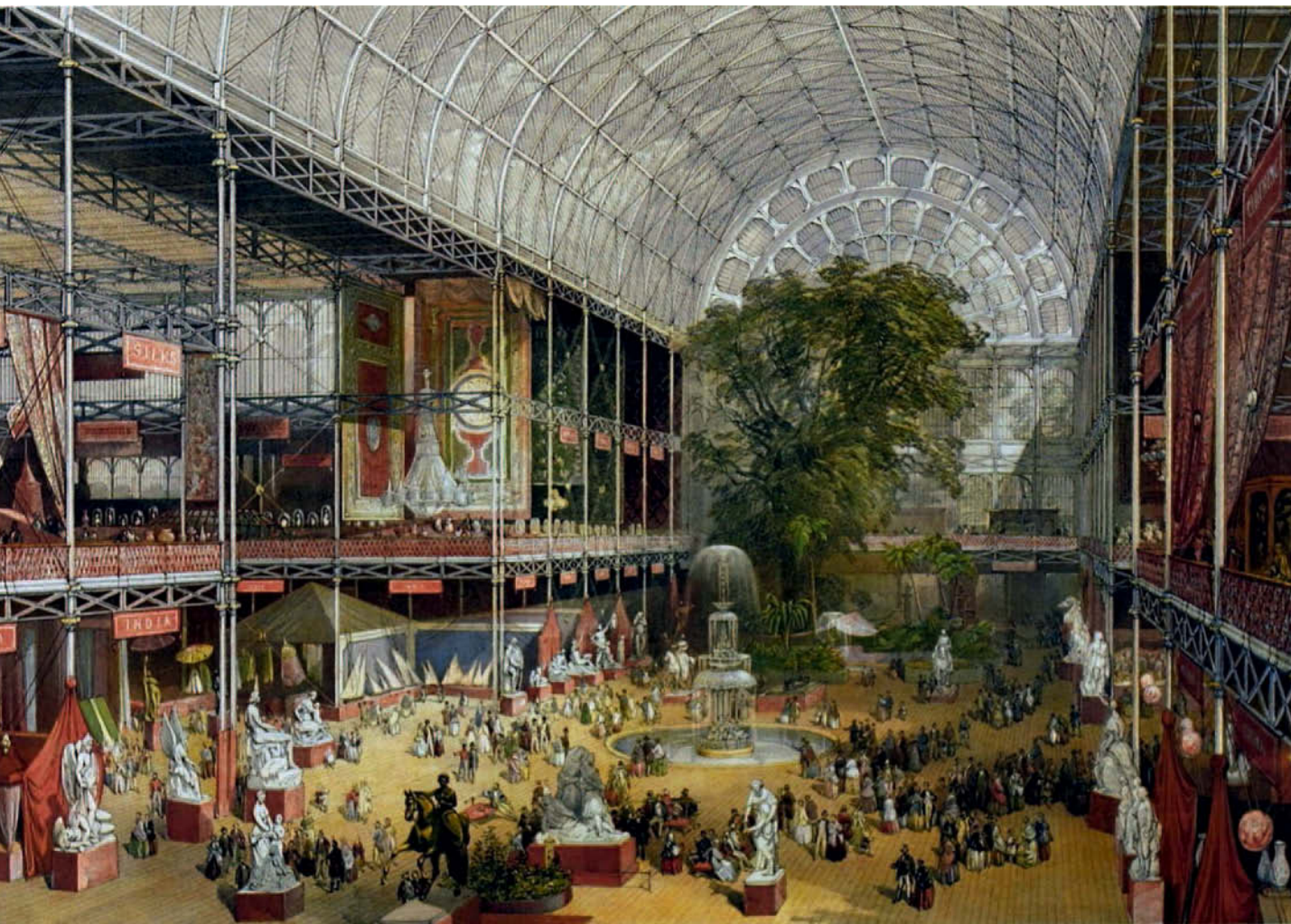
Figure 8.4 The Crystal Palace, London, 1851; Joseph Paxton, designer. It required both a new technology and a purely functionalist approach to design to create this enormous building. Both of these were alien to mainstream architecture of the period, which was largely concerned with the manipulation of images from previous eras. It was, however, the 'new' imagery (i.e. that of the glass-clad framework) created at the Crystal Palace, rather than the functionalist design methodology that produced it, which would serve as one of the architectural precedents for the Modern period.
