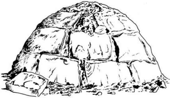
Figure 1.2 The igloo is a self-supporting compressive envelope.
