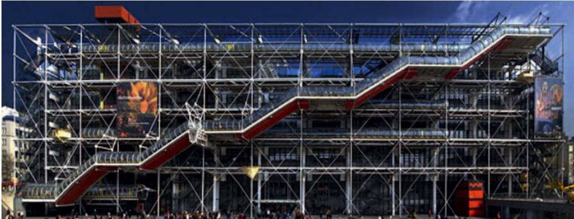
Figure 9.28 Centre Pompidou, Paris, 1978; Piano and Rogers, architects; Ove Arup & Partners (Peter Rice), structural engineers. The Centre Pompidou is perhaps the ultimate expression of ‘techno-optimism’, a celebration of the Modernist belief that the solution to the world’s problems will lie in ever more sophisticated technology.
