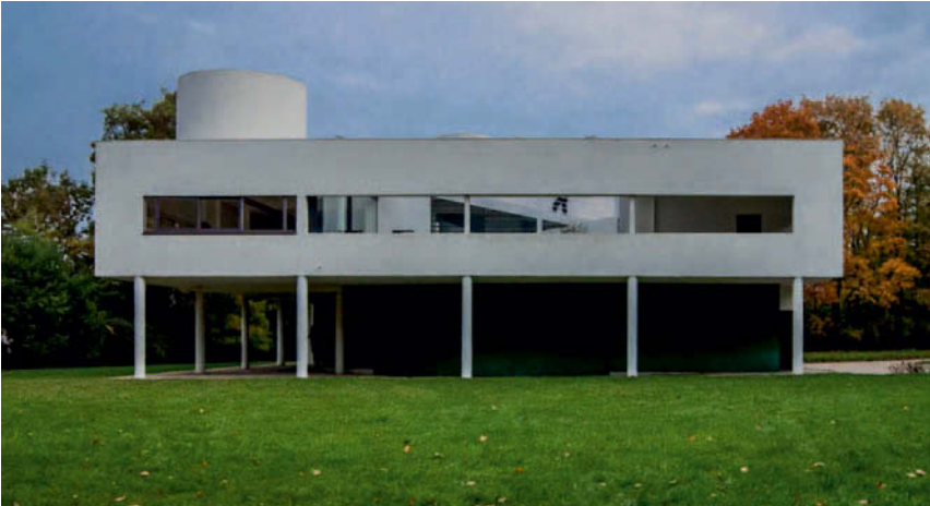
Figure 9.24 Villa Savoye, Poissy, France, 1929; Le Corbusier, architect. Although visually similar to the Highpoint building, the Villa Savoye lacks its constructional integrity. The wall planes here are of non-structural masonry carried on a reinforced concrete frame. Artifice is used to disguise the lack of integration of the architecture and engineering. Photo: Inexhibit/© FLC/ADAGP, Paris and DACS, London 2018.
