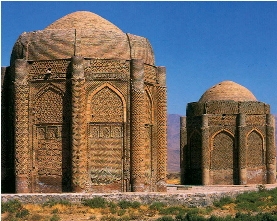
Figure 3.2 Kharraqan Towers, Qazvin, Iran, C11 CE. These 15 m-high late-medieval brickwork structures demonstrate one of the advantages of masonry, which is that very large constructions with complex geometries can be achieved by relatively simple building processes.
