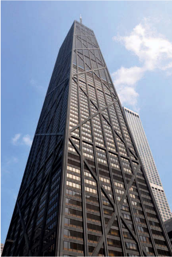
Figure 10.14a John Hancock Building, Chicago, USA, 1969; Skidmore, Owings & Merrill, architects and structural engineers. The trussed-tube structure here forms a major component of the visual vocabulary.
