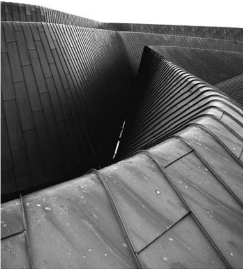
Figure 10.26 Riverside Museum, Glasgow, 2011, Zaha Hadid, architect; Buro Happold Engineering, engineers. The continuous variation in width and depth of the ridges and furrows of the roof greatly complicated the detailing of the supporting steelwork (see also Figure 1.11).
