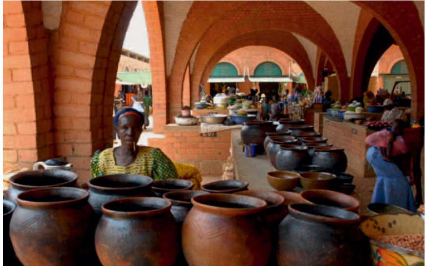
Figure 11.13 Central Market complex, Koudougou, Burkina Faso, 1999–2005; Swiss Agency for Development and Cooperation, architects and project directors. This complex, which involves 85 domes, 658 vaults and 1,425 arches covering a total area of 29,000 sq m (312,000 sq ft) provides shops, commercial accommodation and social spaces in the third largest city in Burkina Faso. It was constructed entirely from locally available materials (principally bricks and blocks in hand-pressed soil) and was designed to minimise solar exposure and enhance air circulation within its large and densely occupied interior. It is remarkable for its combination of low-tech materials and construction methods with a sophisticated approach to design.
