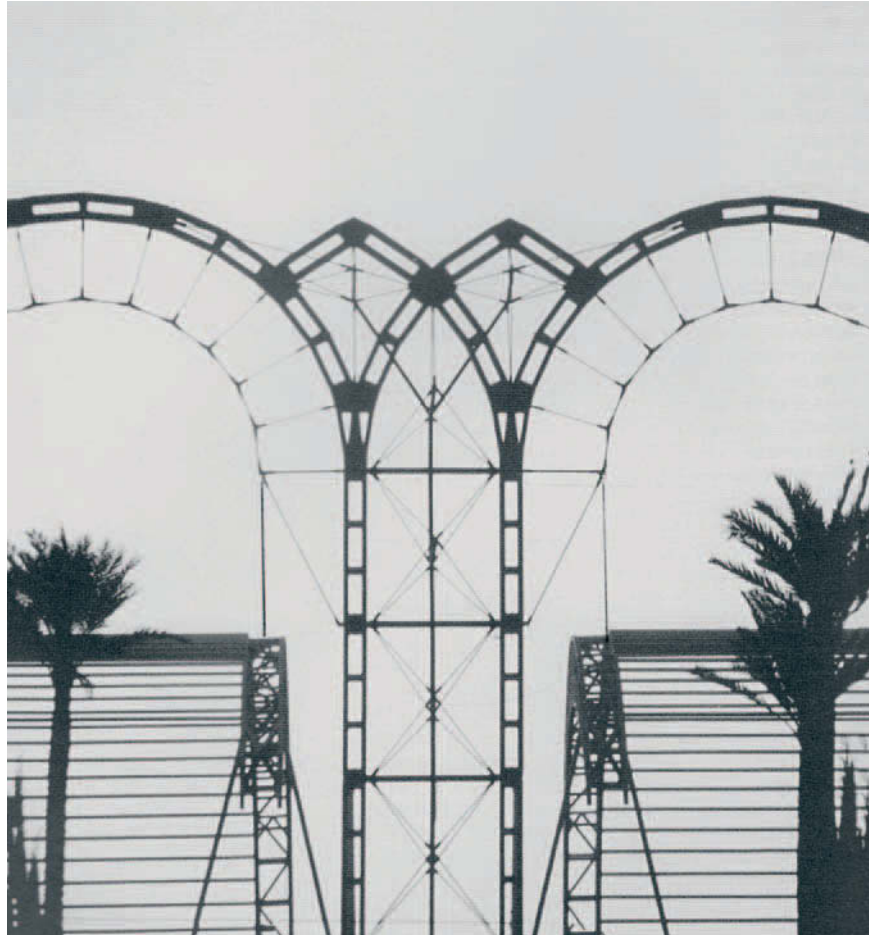
Figure 11.16 Pavilion of the Future, Expo 92, Seville, Spain, 1992; Martorell Bohigas Mackay, architects; Arups (Peter Rice) engineers. One of the structural walls of this building consisted of a composite of slender steel elements and stone masonry blocks. The perfectly plane surfaces of the machine-cut stone blocks allowed smooth transfer of load without bedding in mortar. The filigree steelwork was arranged to apply the load to the masonry arches such that they were subjected to pure axial compression (form-action). The structure was intended as a demonstration that, with the use of contemporary shaping techniques, stone masonry might be reconsidered in the future as a structural material.
