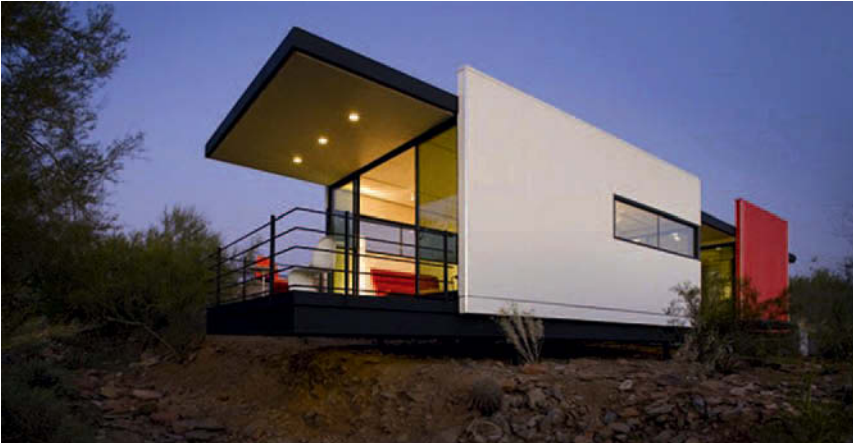
Figure 11.4 Taliesin Mod.Fab House; Taliesin-West-Studio, architects. The cantilevering of the roof and floor planes and the extensively glazed external walls required the use of a structural steel framework for this modest-scale building. The building contains green features, such as off-grid capability and insulated wall panels, but its ecological footprint is considerably greater than required for a building of this size. Stylistic considerations have been given priority over sustainability.
