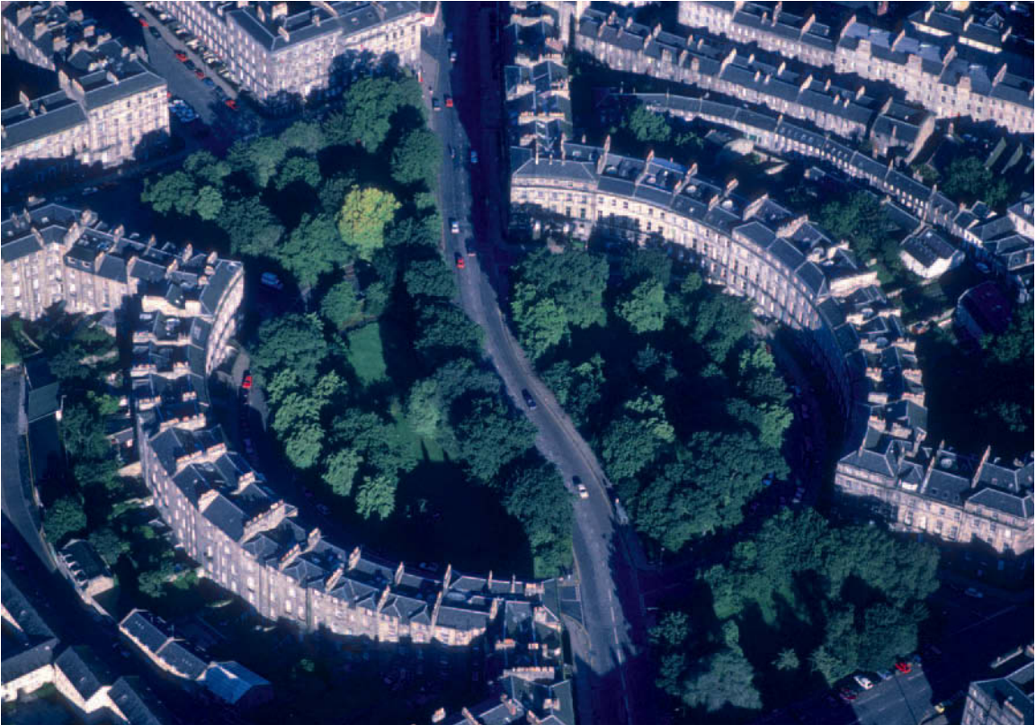
Figure 11.15 Town houses, New Town of Edinburgh, Scotland, c.1800 CE. Buildings such as this, with stone masonry walls and slate-clad roofs, were common throughout Scotland in the pre-Modern period and are examples of a building tradition, based on the use of locally available materials, that was well adapted to the climate of the region. After more than 200 years of continuous use, and with minimal maintenance or adaptation, they still form an important part of the building stock. This truly sustainable architecture, which also performs well in relation to the criteria of good structural design articulated by Nervi and Torroja (see Section 8.2), with suitable incorporation of contemporary technology, could provide one type of precedent for the sustainable built environment of the future.
