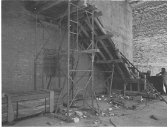
Strutting to the Sloping Soffit Form
