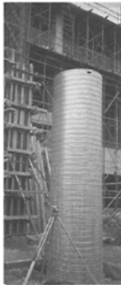
Spirally Wound Proprietary Column Form
