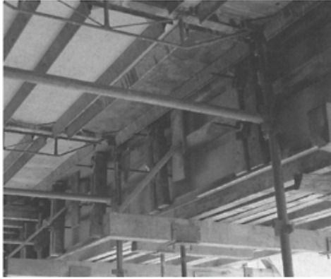
Proprietary Quick Strip Soffit Form System
