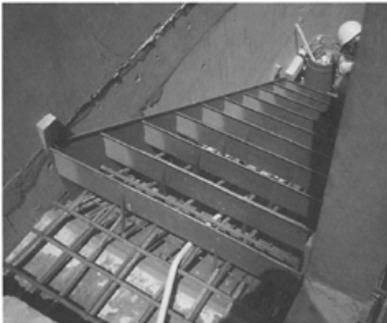
Sheet Metal Stair Form in Place
