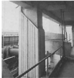
Precast Forms to all Column Faces
