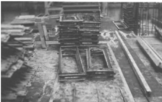
Components Stacked on the Formwork
