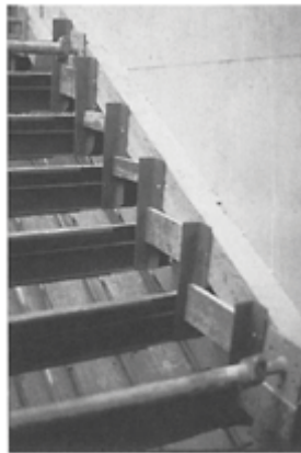
Stair Riser Forms Fixed to Plate on Wall
