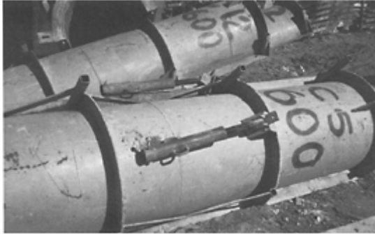
Steel Column Formwork with Bracing Attached.
