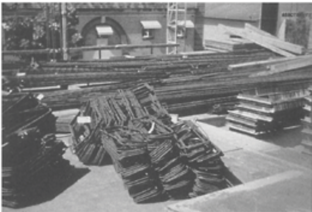
Reinforcement Stacked on the Formwork
