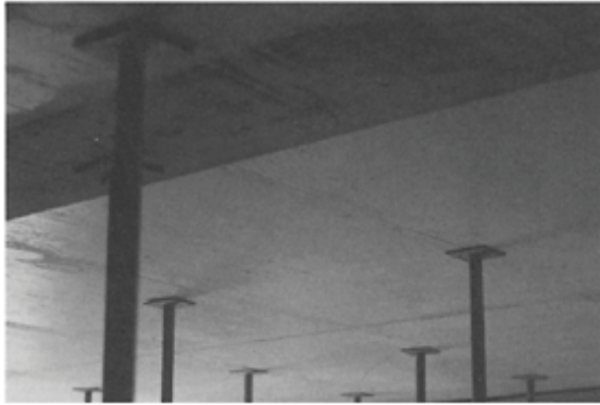
After the Removal of All Formwork Framing and Plywood
