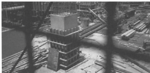
Materials Stacked on Site
