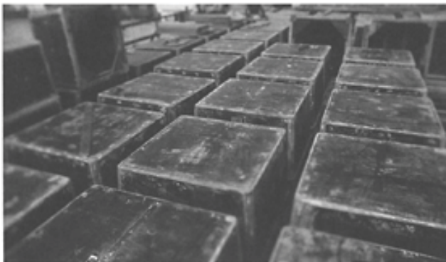
Timber and Plywood Waffle Forms
